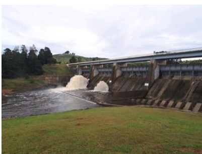
Scrivener Dam over flow. Dairy Farmers Hill in the background
