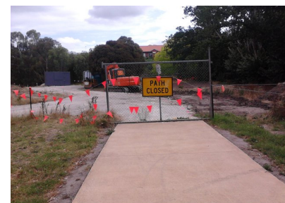
Works have now commenced Boulevard side of bridge
