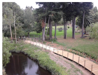
Trail works in progress passing under the Heidelberg Rd bridge
